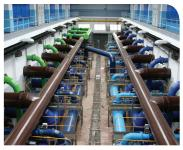
The surface water from AVEK is treated at their treatment plant using conventional treatment methods, which include coagulation, flocculation, sedimentation and filtration. The water is then disinfected to kill any remaining microorganisms, such as bacteria, and reduce the potential for their regrowth in the distribution pipes. The groundwater the District serves is also disinfected with chlorine for
